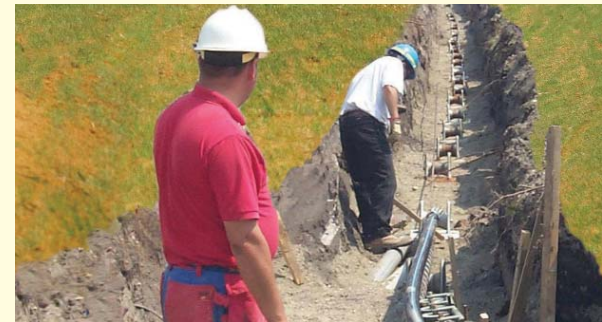
Preparing for trenching
